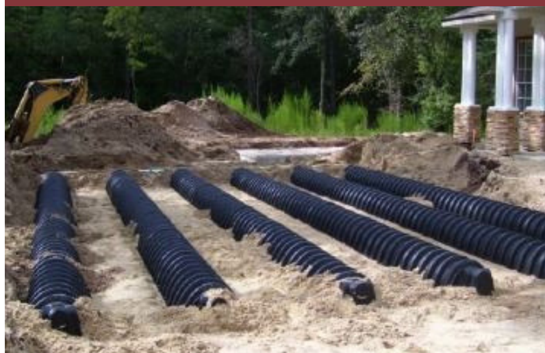
Septic drain field pipes
